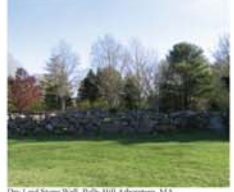
Dry-Laid Stone Wall, Polly Hill, Adirondack, MA
