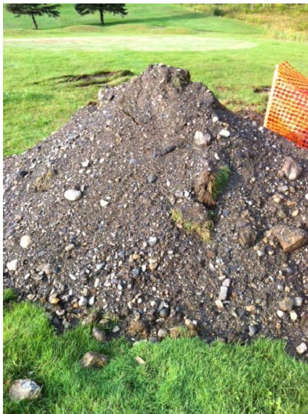
Test Pit DT-4 Spoil Pile
