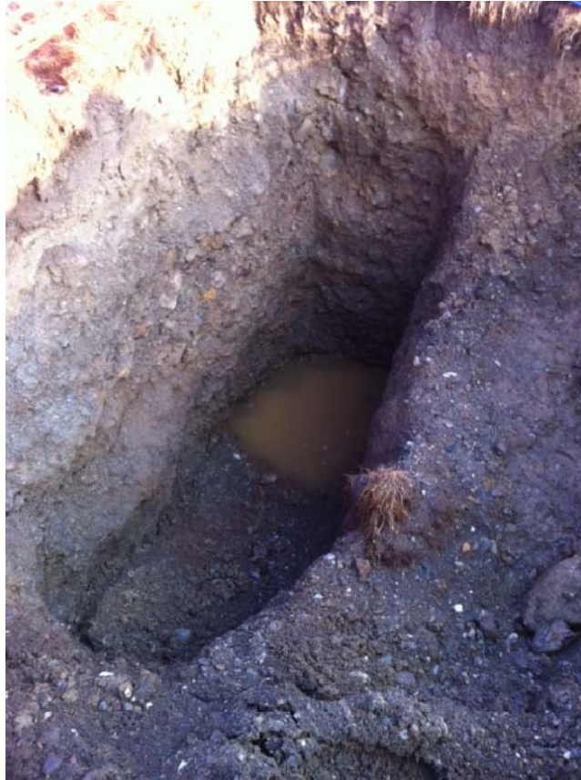
Test Pit DT-2, Note Standing Water
