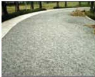
Pervious Concrete Paving
