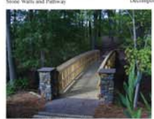
Wooden Footbridge with Stone Piers
